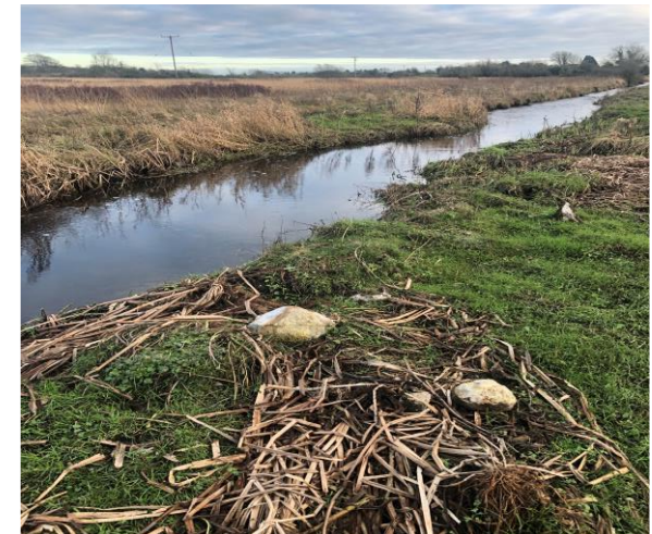
Fig 4. Stones and weed and gravel recently removed from the Nanny R. during drainage maintenance
