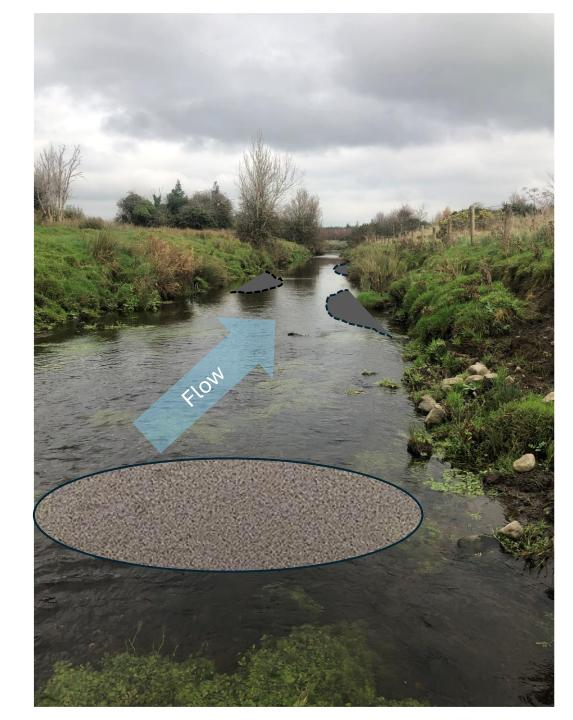
10. From Ch 27060 - 26905 Construct #5 alternating deflectors to narrow base with, increase flow rate and create thalweg.
