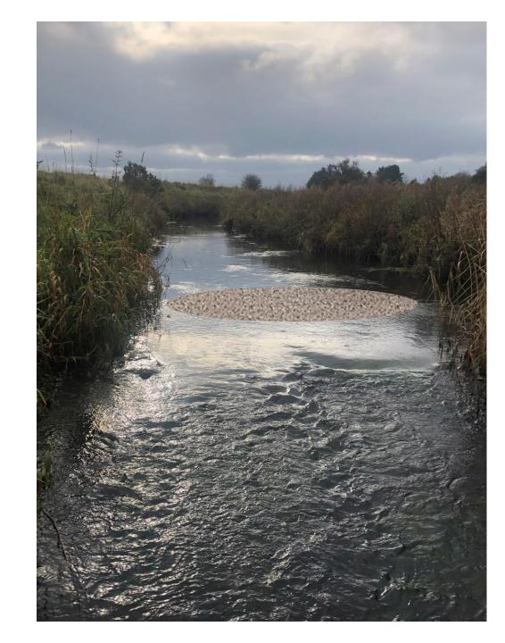
7. Ch27195 Place a gravel bed at the downstream end of the pool on bend.
