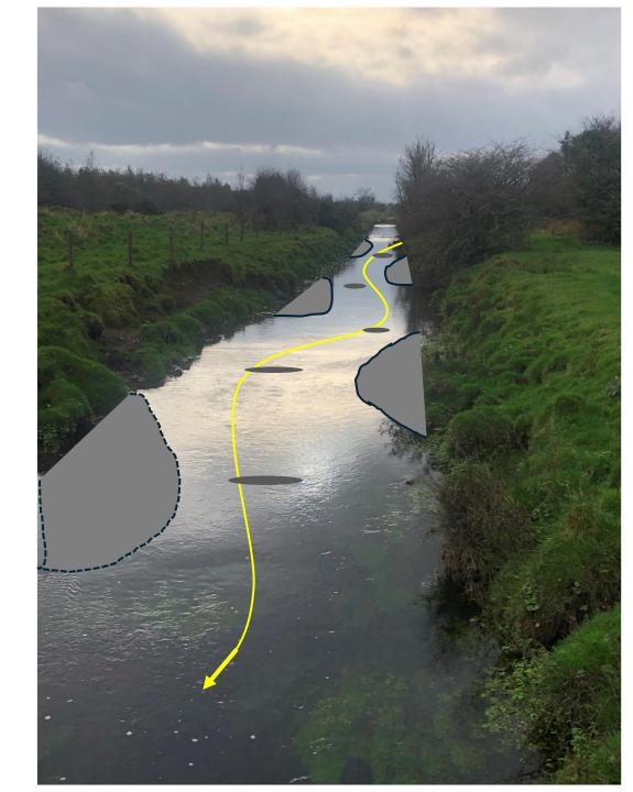
11. Ch. 26910 Place large gravel bed upstream of gradient break at last riffle upstream of footbridge Fence entire length of left bank for this stretch. (C. 230m)
