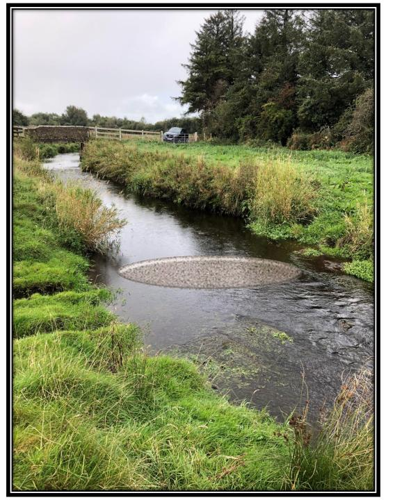
1. Chainage 27670. Place gravel bed (approx. 5T) at tail end of pool 20m downstream from bridge
