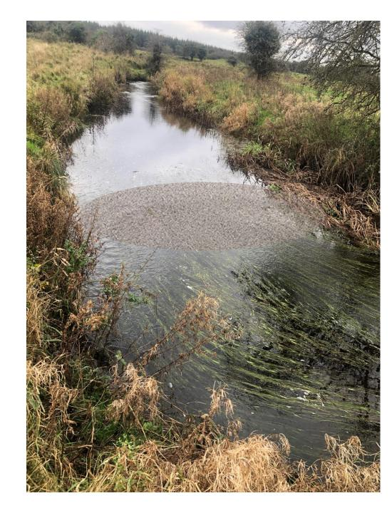
9. Ch 27065 Place large gravel bed 2m upstream of riffle
