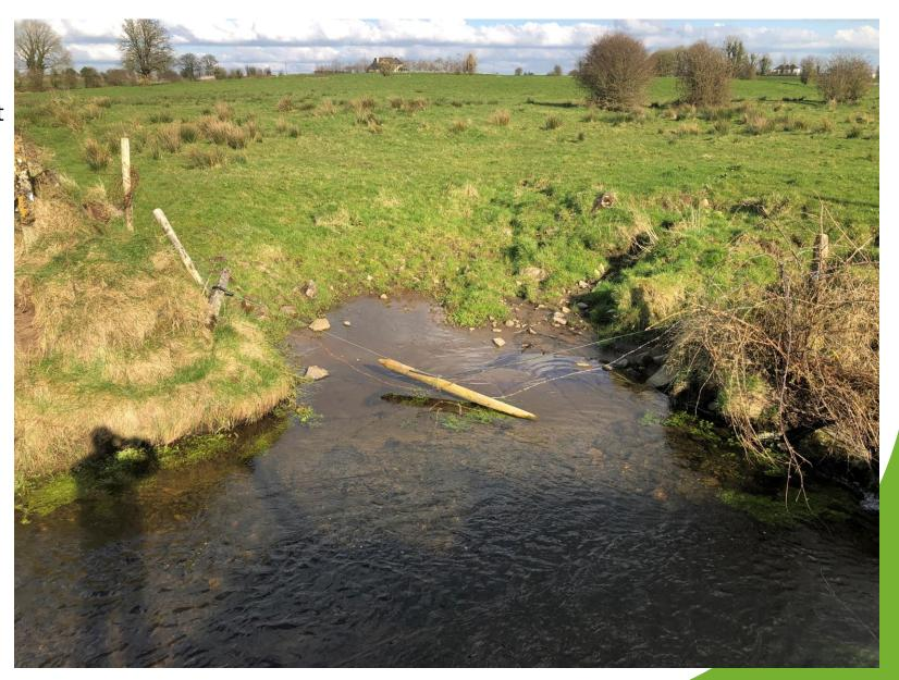
Ch 840. Place large gravel bed (6T), 2m upstream of gradient break at end of existing pool
