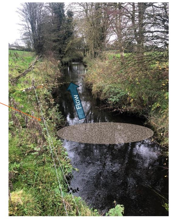
2. Ch23870 – Place Gravel bed (C. 3T) at gradient break as shown here
