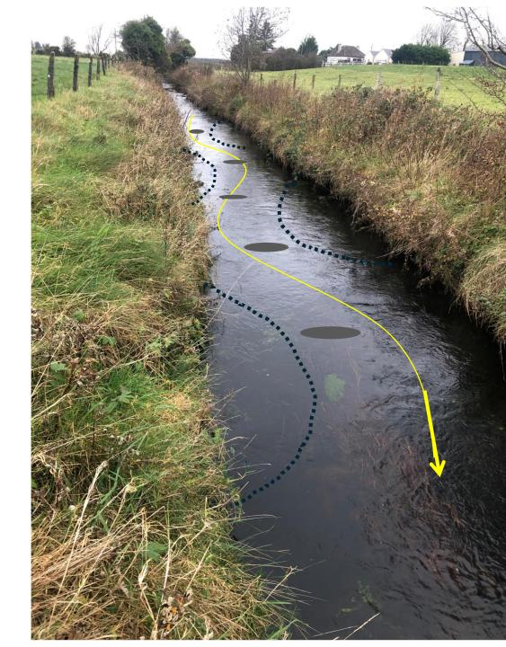
Ch. 24240 Place Gravel bed (C. 3T) at gradient break as shown here
